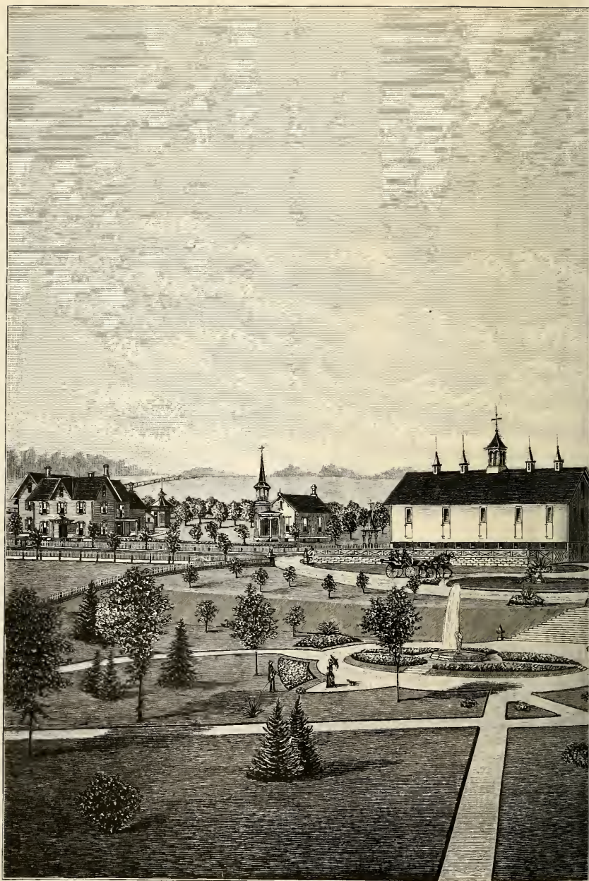
“SU RESIDENCE OF SWATARA TOWNSH
